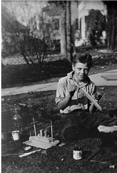
Figure 10. The front yard workshop, while school was closed for influenza. Mountain Division, Denver, CO, 1919. (Library of Congress. Local Identifier: 2017668474)
